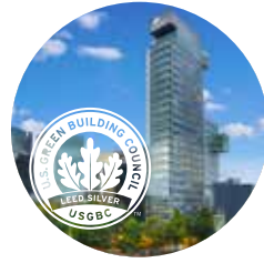
Torre IOS OFFICES
