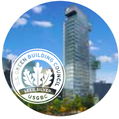
Torre IOS OFFICES
